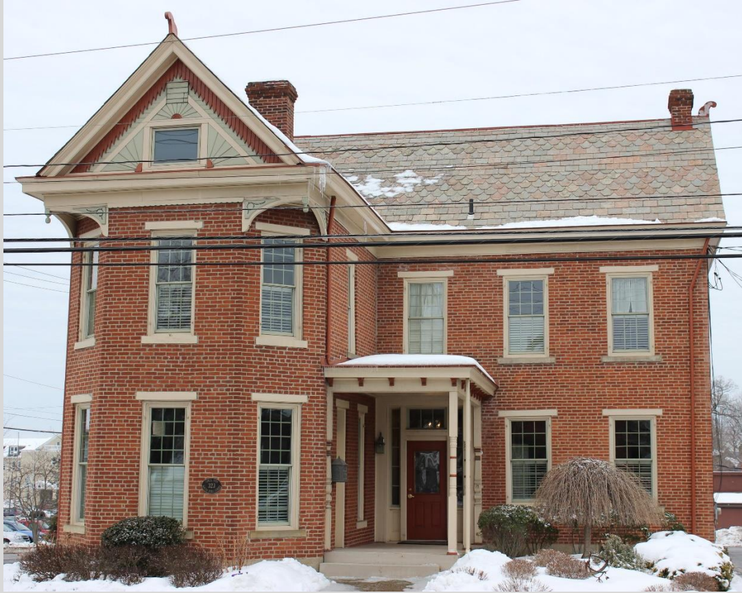
1854 Muntz House at 323 S. Main Street
