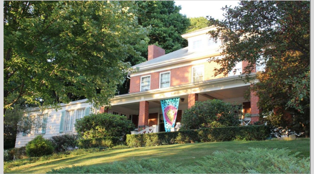
Duffmont – along South Main Street
